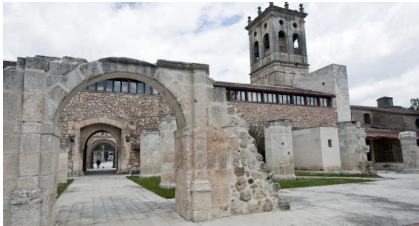
Interior space of the complex of building
